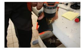
Insert the switch to the hole, connect the cables, and install the console (now with the 3-way switch) back to its place.
